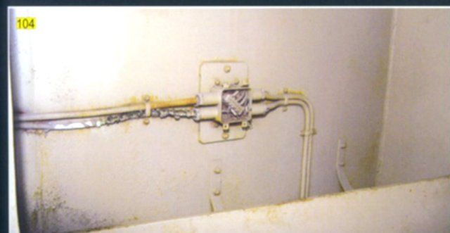
104 105 Examples of rather incomplete fuse and switch boxes. They would have had lids originally.
